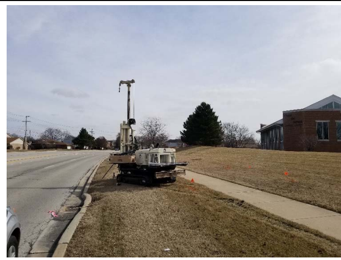
Photograph 8: Advancement of B7, facing northeast
