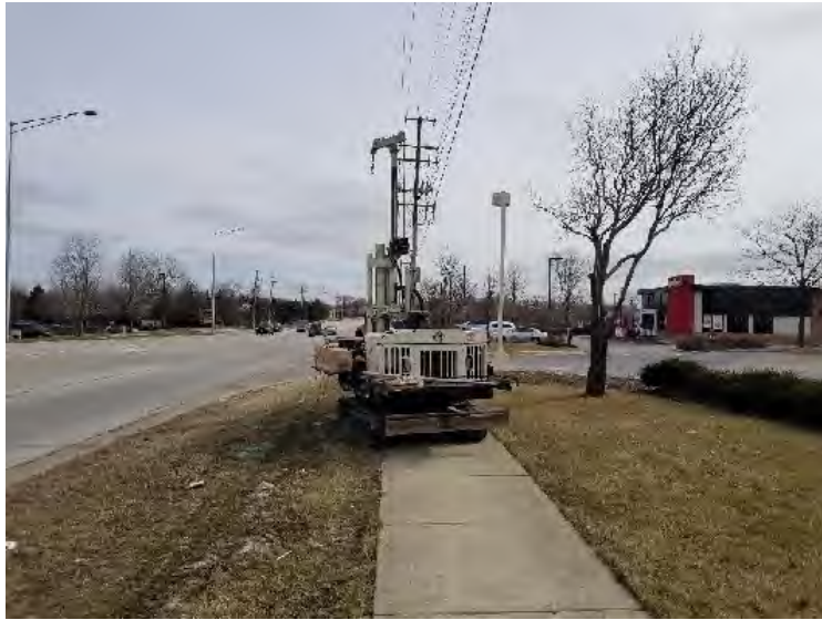
Photograph 5: Advancement of B5, facing east
