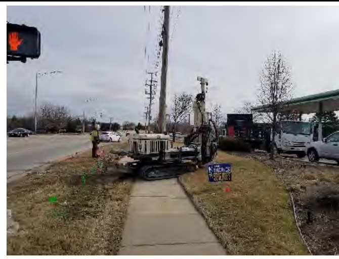
Photograph 4: Advancement of B4, facing east
