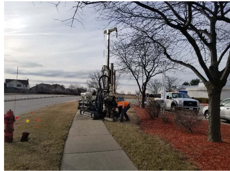
Photograph 2: Advancement of B2, facing east
