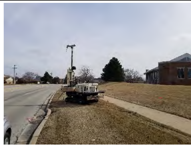
Photograph 8: Advancement of B7, facing northeast
