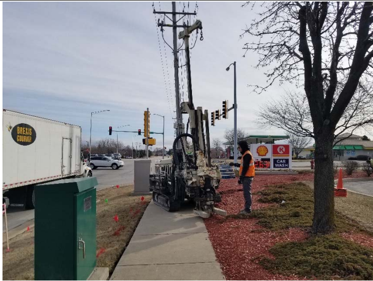
Photograph 1: Advancement of B1, facing east
