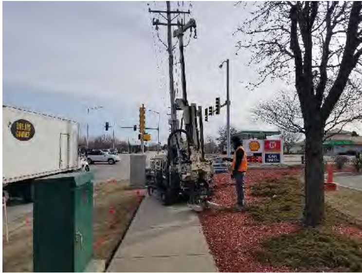
Photograph 1: Advancement of B1, facing east
