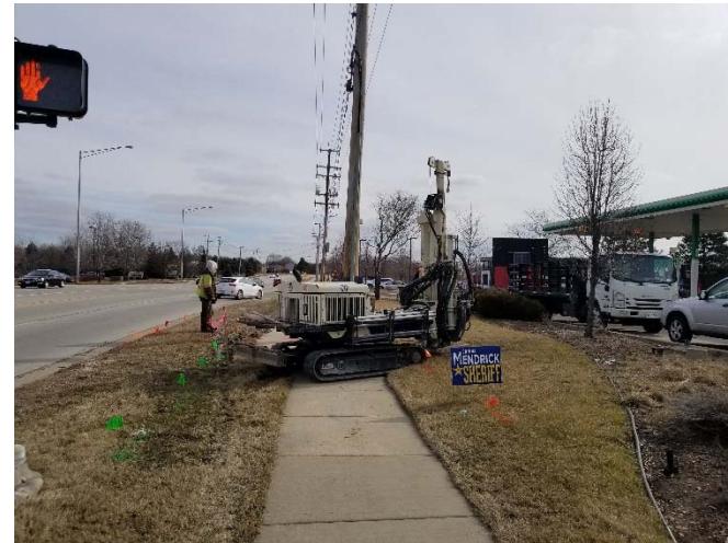
Photograph 4: Advancement of B4, facing east
