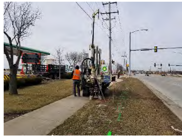
Photograph 6: Advancement of B5, facing west
