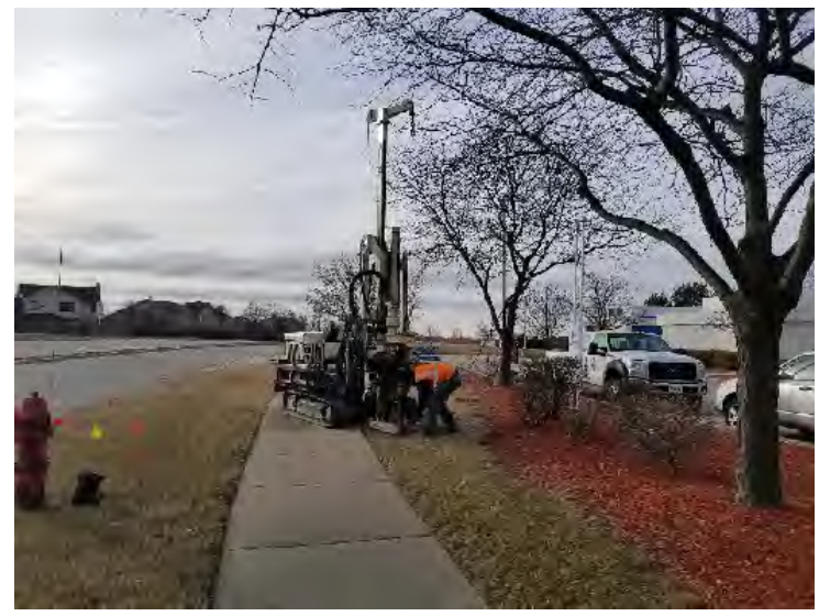
Photograph 2: Advancement of B2, facing east
