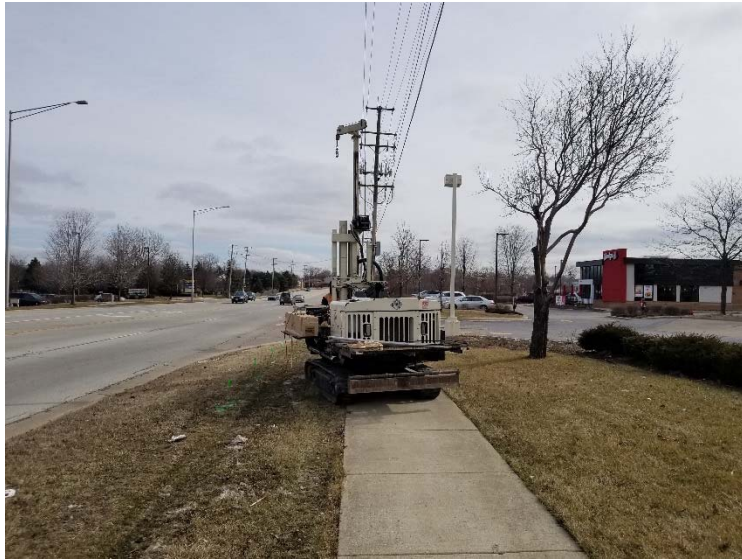
Photograph 5: Advancement of B5, facing east
