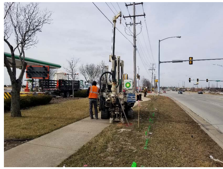
Photograph 6: Advancement of B5, facing west
